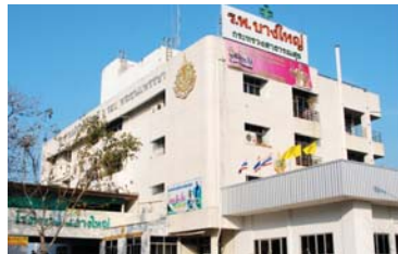
Bangyai hospital : a 30 bedded hospital
